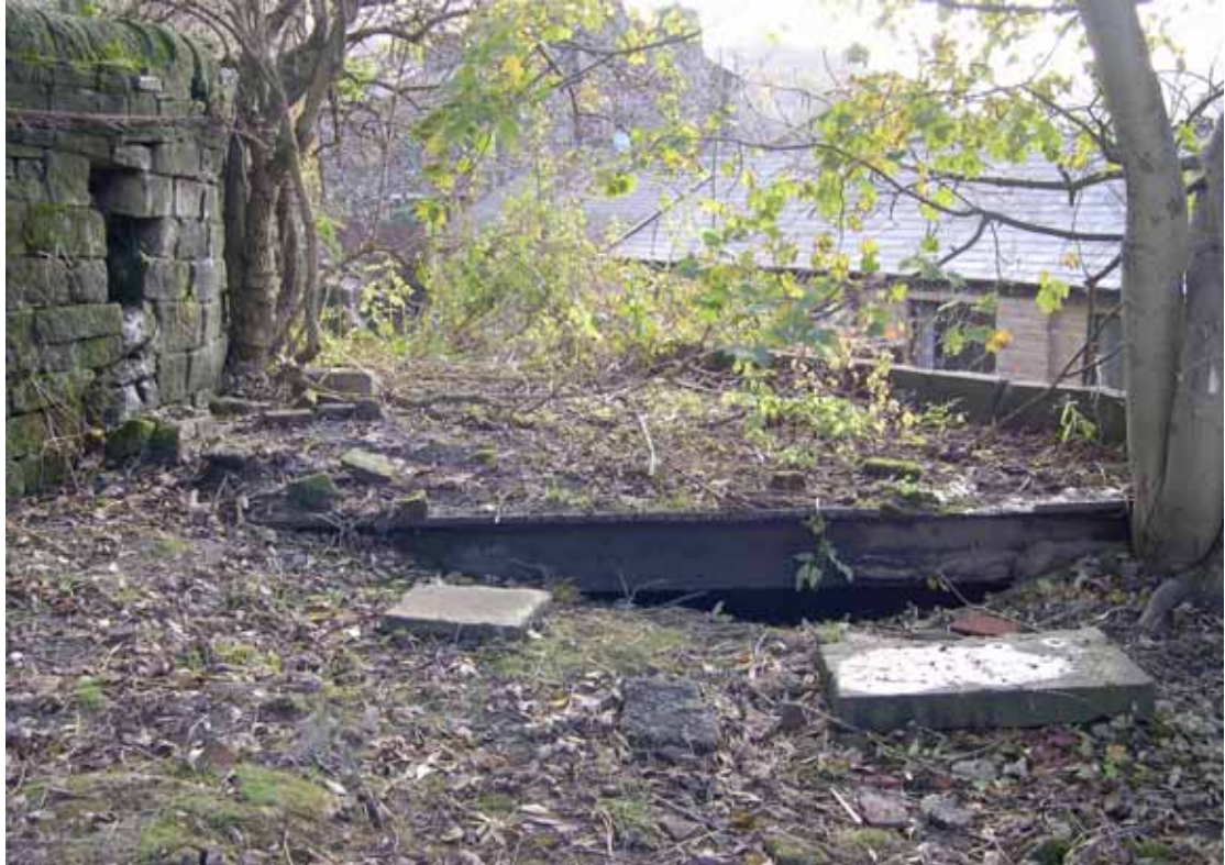
Culvert at apex
