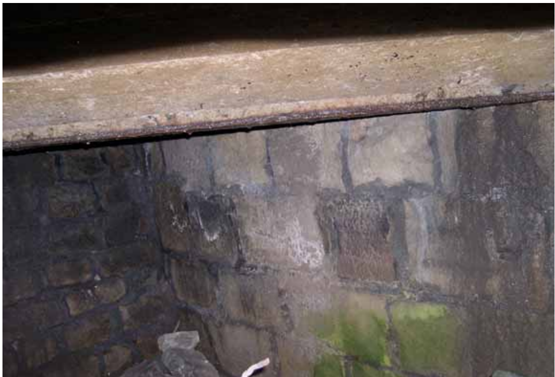
Concrete beam bracing millpond walls at apex
