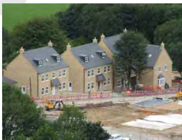
Picture 2.12 New housing development at Fountain Head
